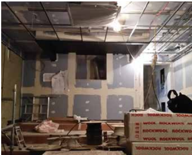
Screening room under construction
